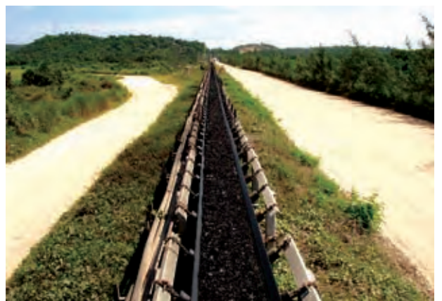
Transporting clean coal to coal blending stockpile.
